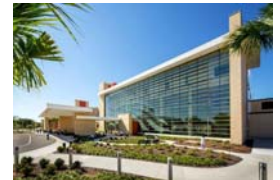
Tampa Polytrauma and Rehabilitation Center
